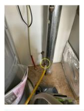
Seismic Straps Installed Not Present
